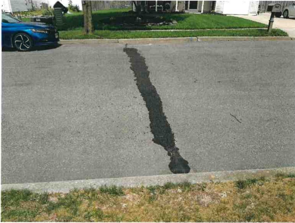
Crack Sealing (typical) along the full width of Spruce Circle North throughout the project area.
