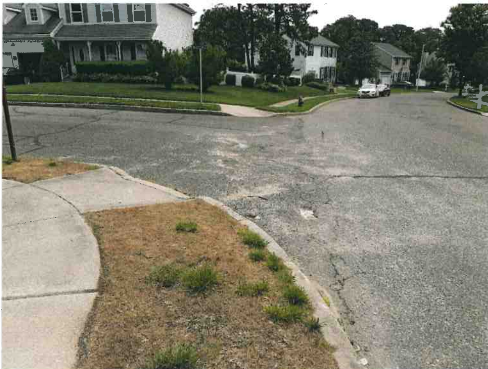
Intersection showing roadway failure.
