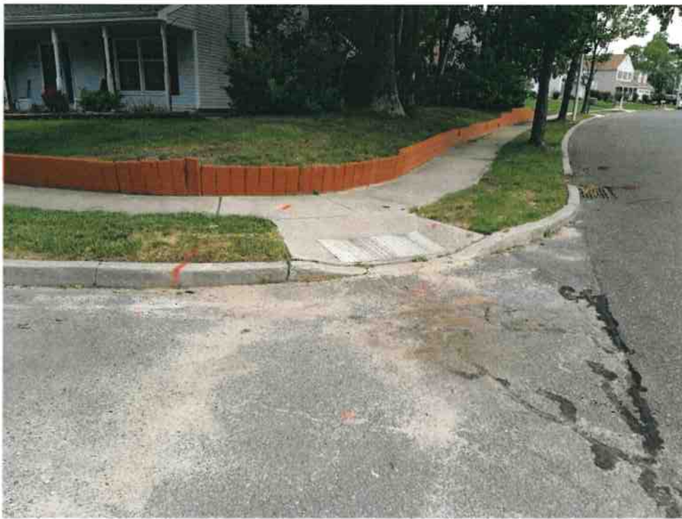
Intersection corner showing road fatigue. Sediment on roadways shows poor drainage. Crack seal repairs found
