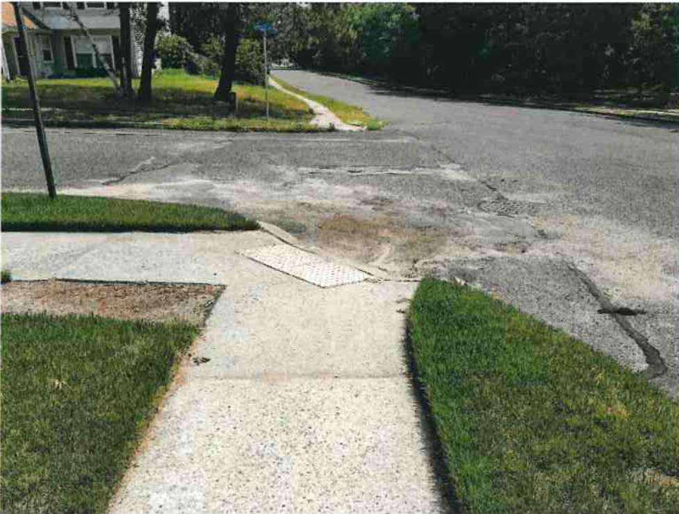
Existing sediment is a sign of poor drainage. Roadway failure and crack seals present.
