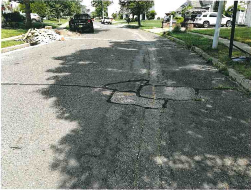
Existing Trench Repair for gas line.
