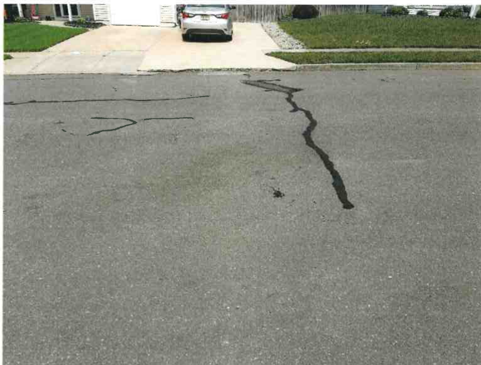
Crack Sealing (typical) on roadway. Concrete Apron is damaged at roadway edge and needs repair.
