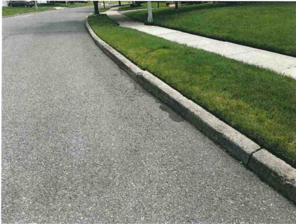
Edge Cracking with crack sealing.
