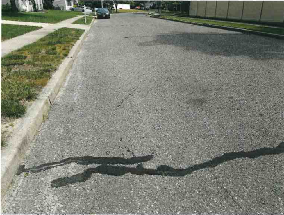
Transverse Cracking is found. Cracks were sealed.
