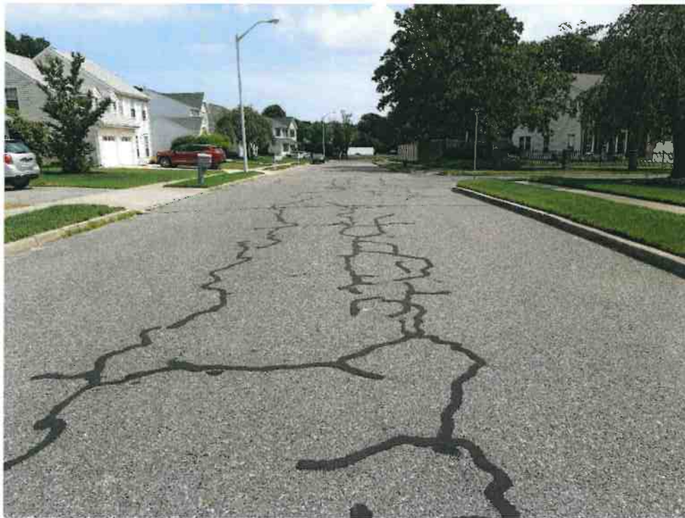
Crack Seal on existing Block Cracks.
